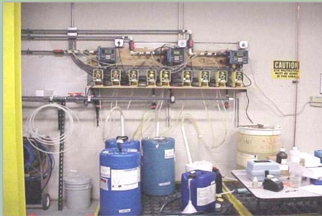
Cooling tower installation using traditional liquids.
