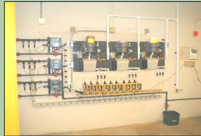
Cooling tower installation using solid Chemical Treatment.
